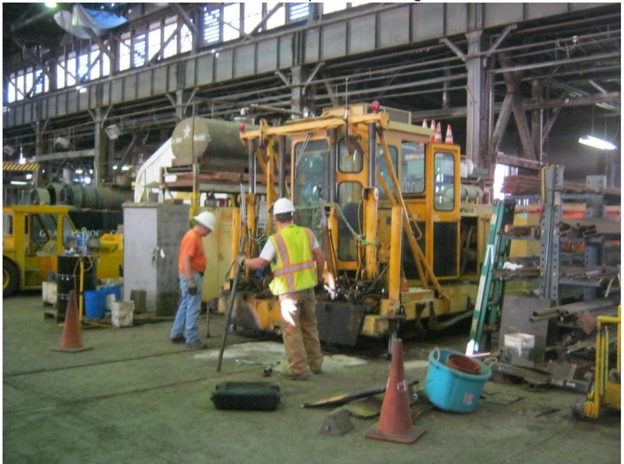
Mike H. and DJ work to remove the work-head sliders from the "new-old" tamper
