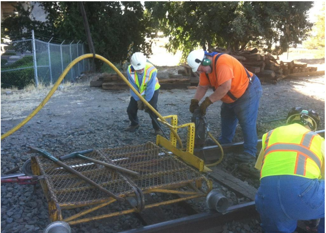
Mike M., Frank, and Mike F. spiking using Alan's new spiker trolley and air hose caddy.
